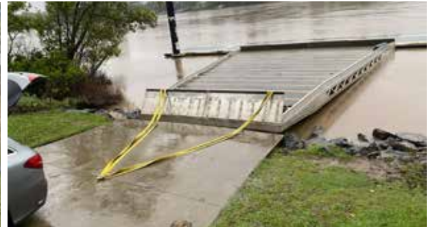
Pontoon Repairs Underway
